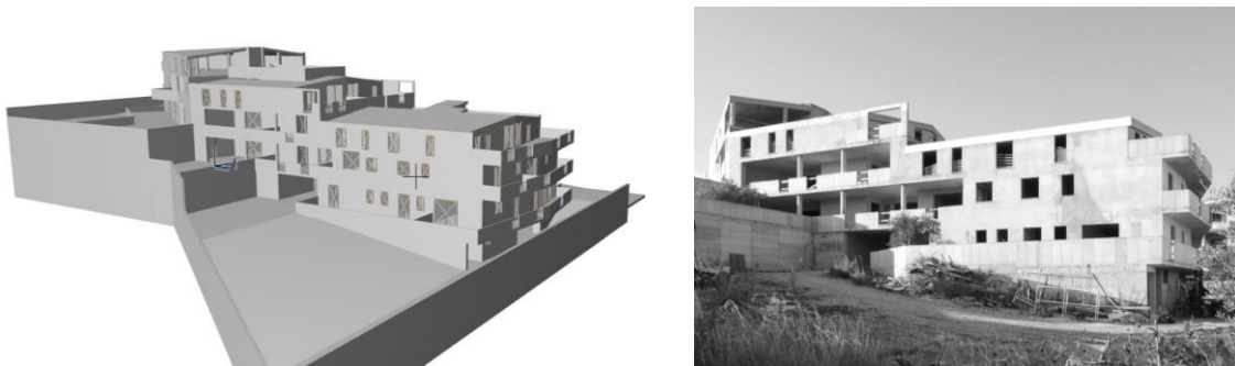
Figure 4-1 San Salvo - Italian demo site. BIM (left) and north-east view (right).
