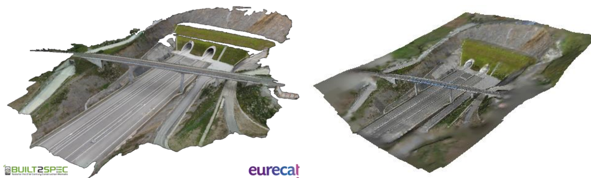
Figure 3-5 3D reconstruction of the viaduct done by Eurecat (Pix4D, left) and by ETH (COLMAP, right).
