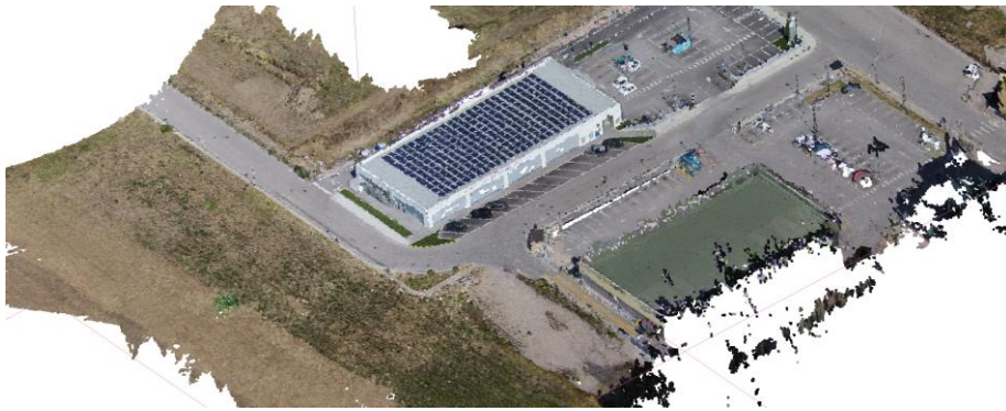
Figure 4-17 BIM and 3D reconstruction from drone images acquisition.
